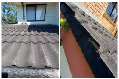
Roof Flashing - Type And Flashing material is of preformed aluminium. Flashings appear to be in serviceable Condition: condition.
